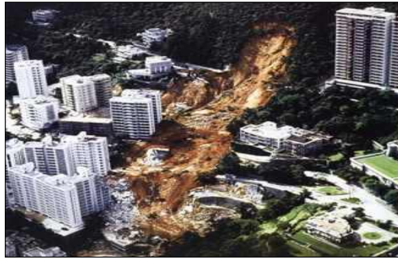
Figure 4. Hong Kong, Po-Shan Road landslide in 1972, presenting the danger of unstable ground conditions, (Photo by Geotechnical Control Office, Hong Kong Government), (Schuster & Highland, 2007).
